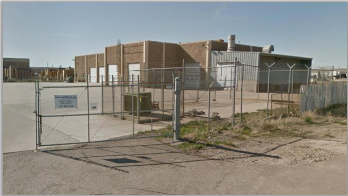
Figure 22. Existing building to be retrofitted as a Bus Maintenance Workforce Training Facility
